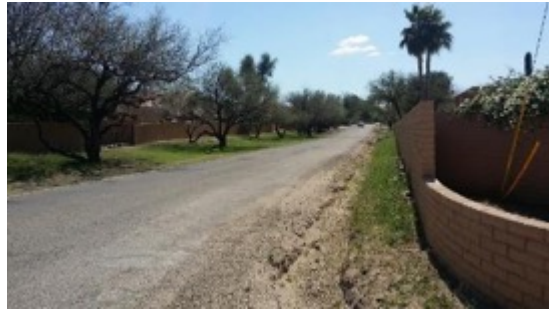
Stormwater detention - Meadow View trench
