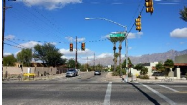
Pedestrian /ADA access - Prince at Tucson Blvd.
