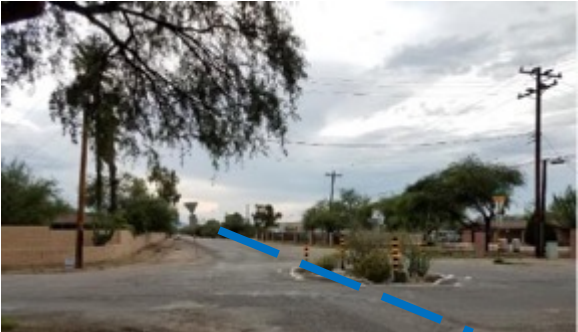
Tie-in to the re-claimed water line in Allen Road for right-of-way landscaping irrigation
